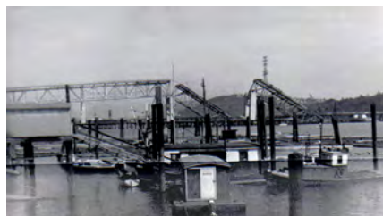
View of the collapsed spans of the Second Narrows Crossing Bridge in August 1958, two months after the collapse. Credit: Ron B. Thompson, Wikipedia, CC BY-SA 3.0
