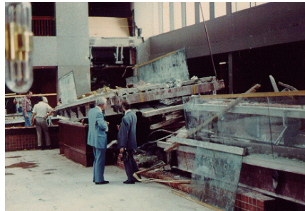
The Hyatt Regency walkway collapse in Kansas, Missouri, killed 114 people and injured 216. It was one of the deadliest structural failures in the U.S. until the collapse of the World Trade Center. Credit: Dr. Lee Lowery, Jr., P.E., Wikipedia, Public Domain.
